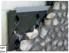
Additional tie, fixed through the pod using a seal -washer
